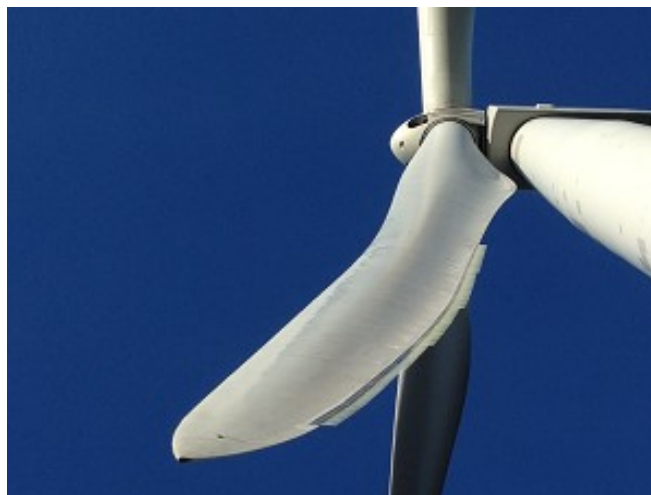
Fig. 1: LNTes at the wind turbine rotor blade
