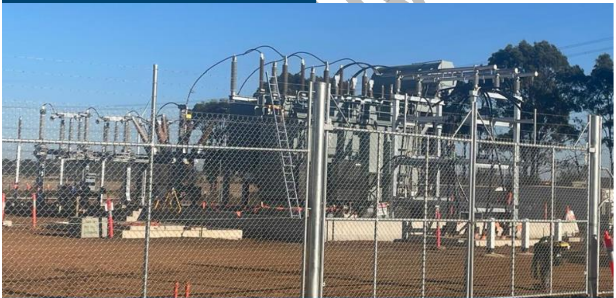
33kV Over head bus installed, 33kV secondary and 132kV primary cables being installed
