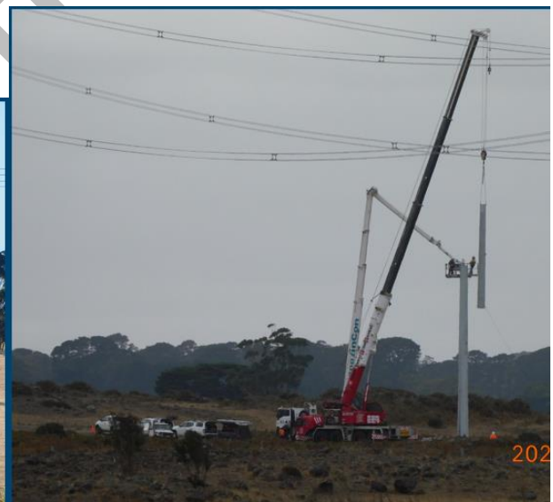
Section 3 being lifted
