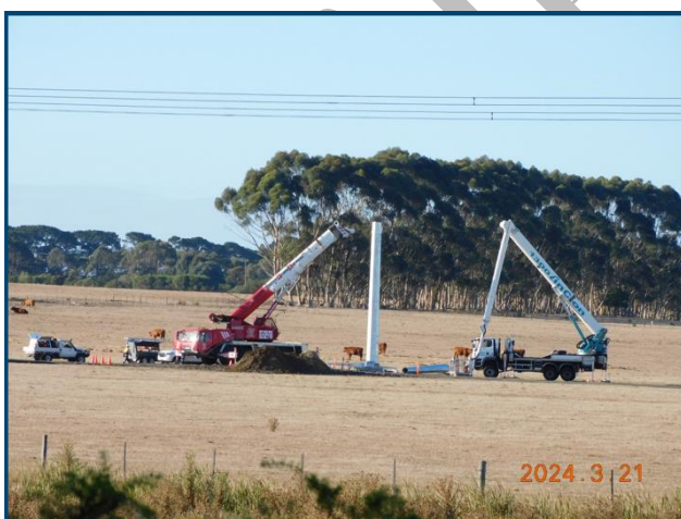
Standing up the first of 3 sections for a transmission pole
