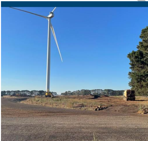
Remediation works underway
