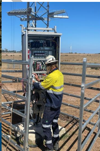
Met mast communications being installed
