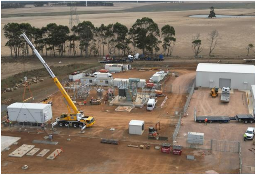
Switch room being positioned
