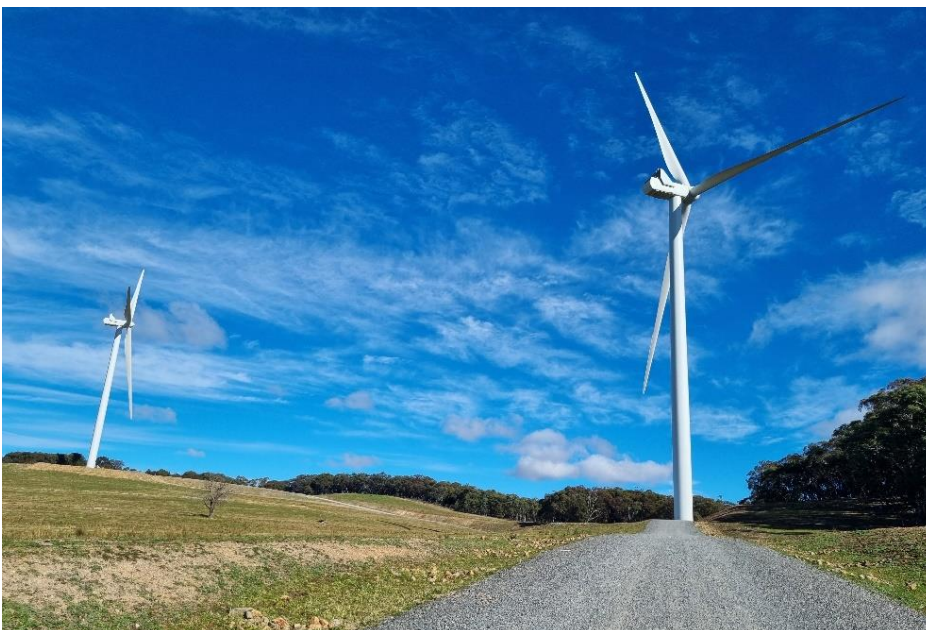
Some turbines at Crookwell Windfarm 3 spinning
