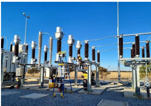
Electrical works being finalised in the Substation
